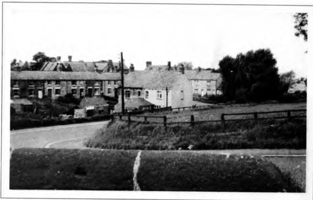
View of the village in 1959 showing the site of the present Meadows Estate
