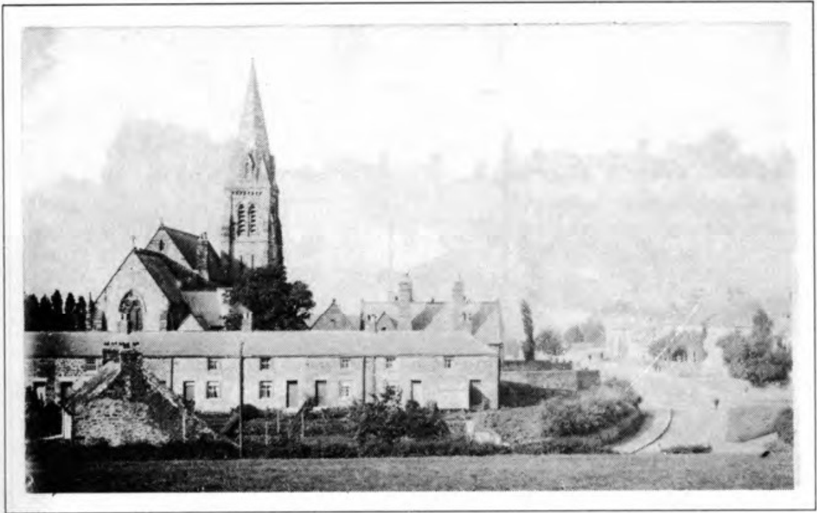
View of the village in 1929 showing the site of the present Meadows Estate
